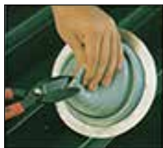
Step One Trim Trim opening to 20% smaller than pipe diameter.
