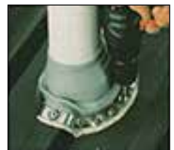
Step Five Fasten Use fasteners to finish sealing.
