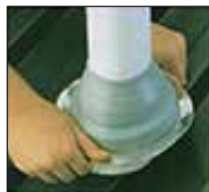
Step Two Slide Slide down over pipe.
